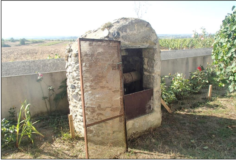
Figure 100 - Puits riverain P3
